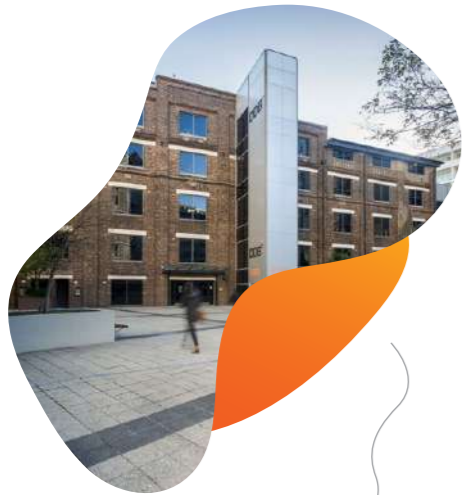
Ultimo Campus 46-52 Mountain St, Sydney
